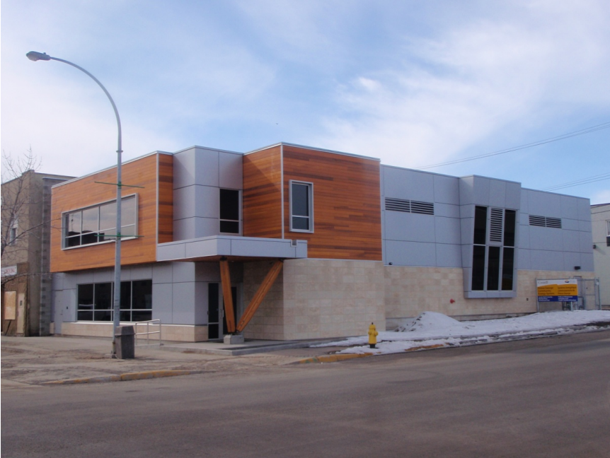
The back-up heating plant for the Downtown District Energy System. (Photo courtesy Adrian Mohareb)
